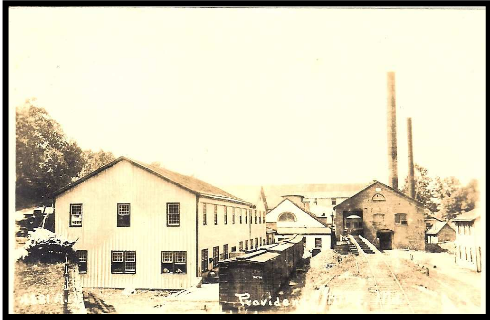
Figure 4. Providence Mill, the end of the line, about 1912
